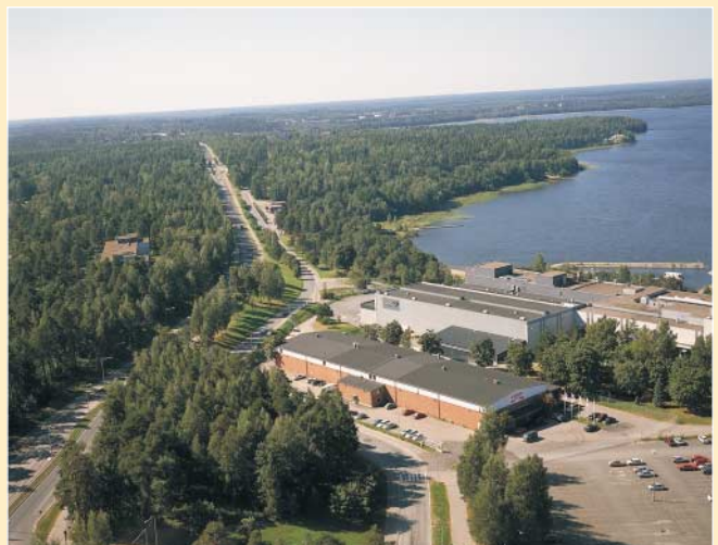
Larox is investing significantly in its new business premises in Lappeenranta, Finland.
